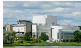
Finish National Opera, Helsinki
